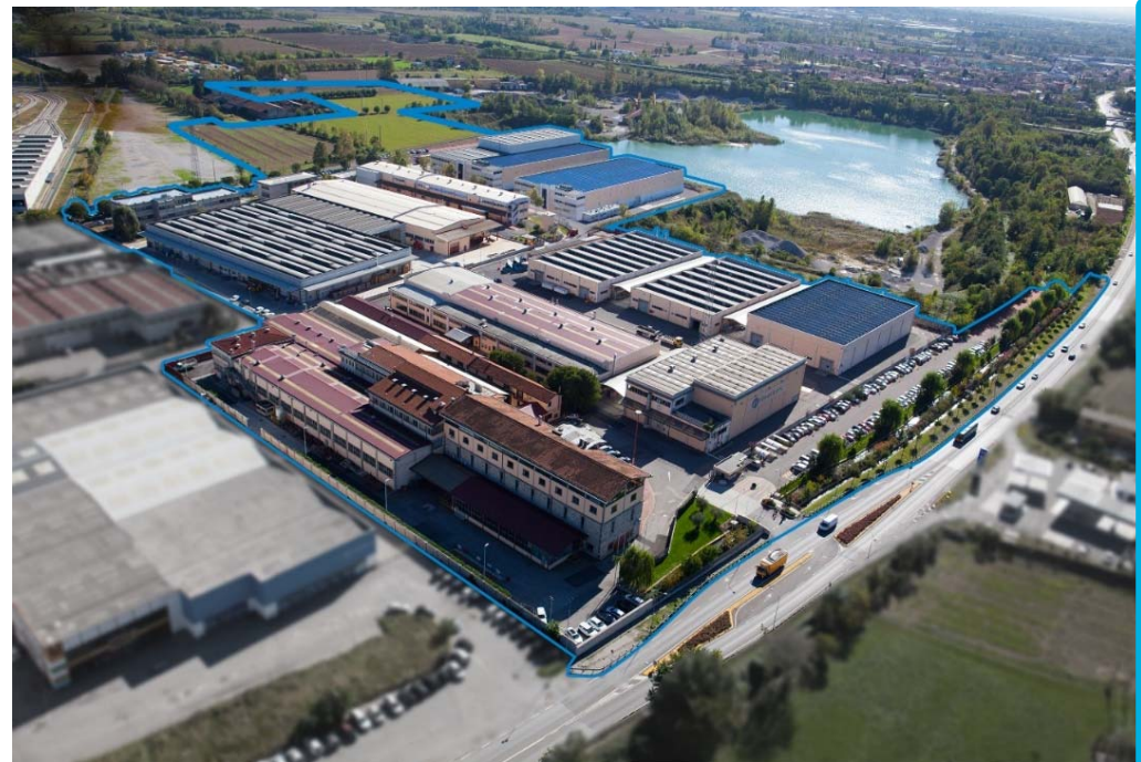
CEMBRE S.p.A. – Headquarter in Brescia (Italy)
