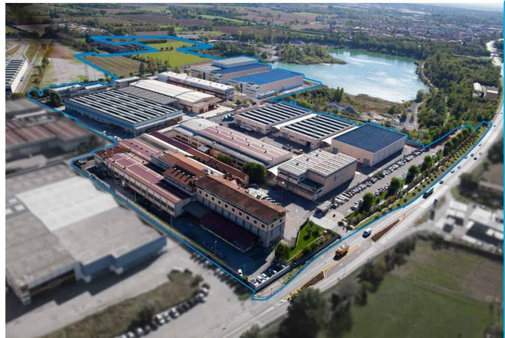
CEMBRE S.p.A. – Headquarter in Brescia (Italy)
